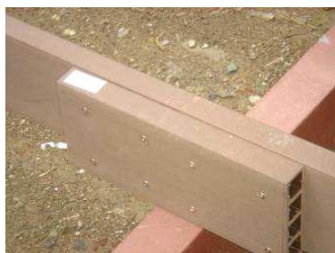
Add one more joist
